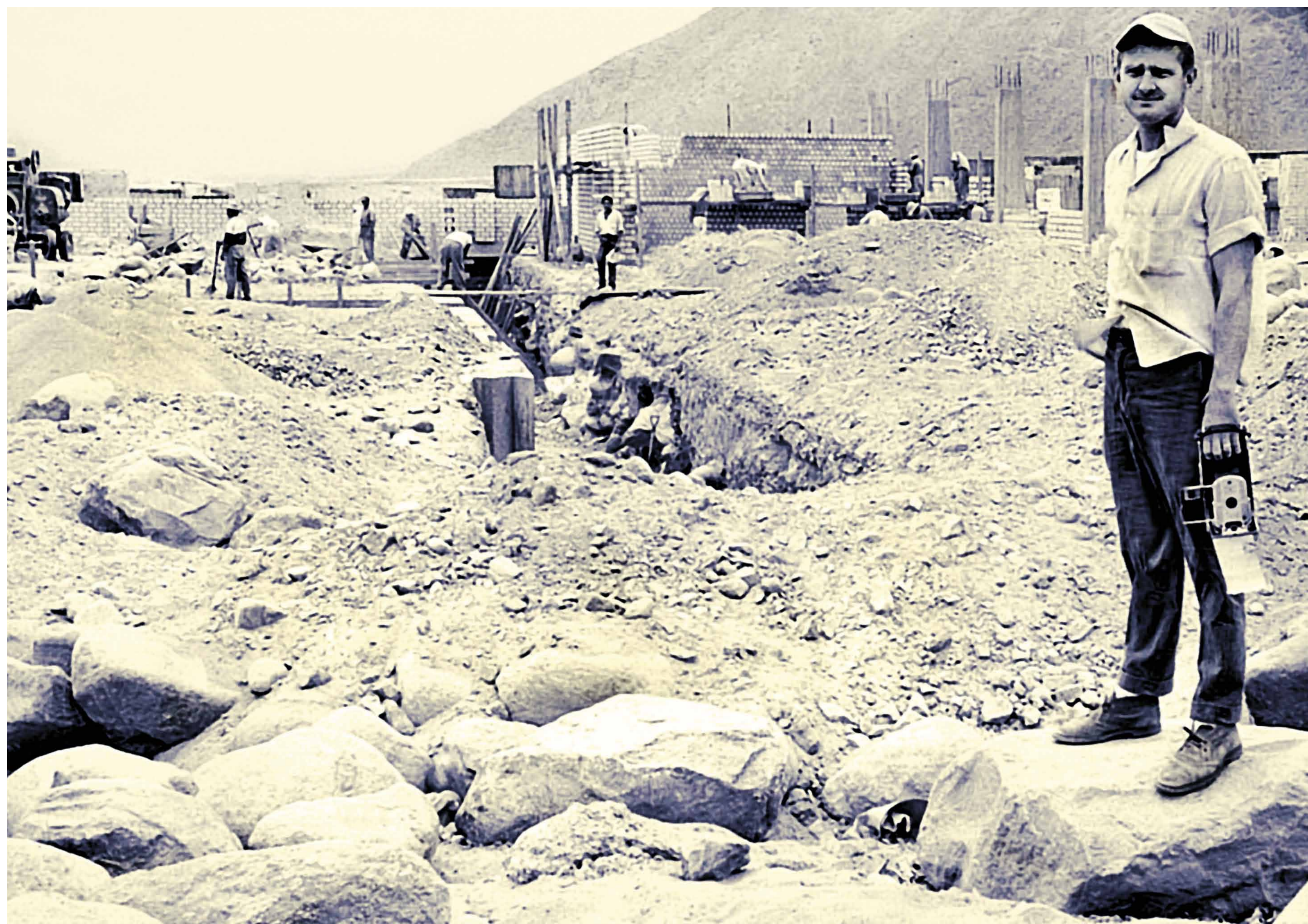
Start of construction: Ben checking building construction progress. (1961)
