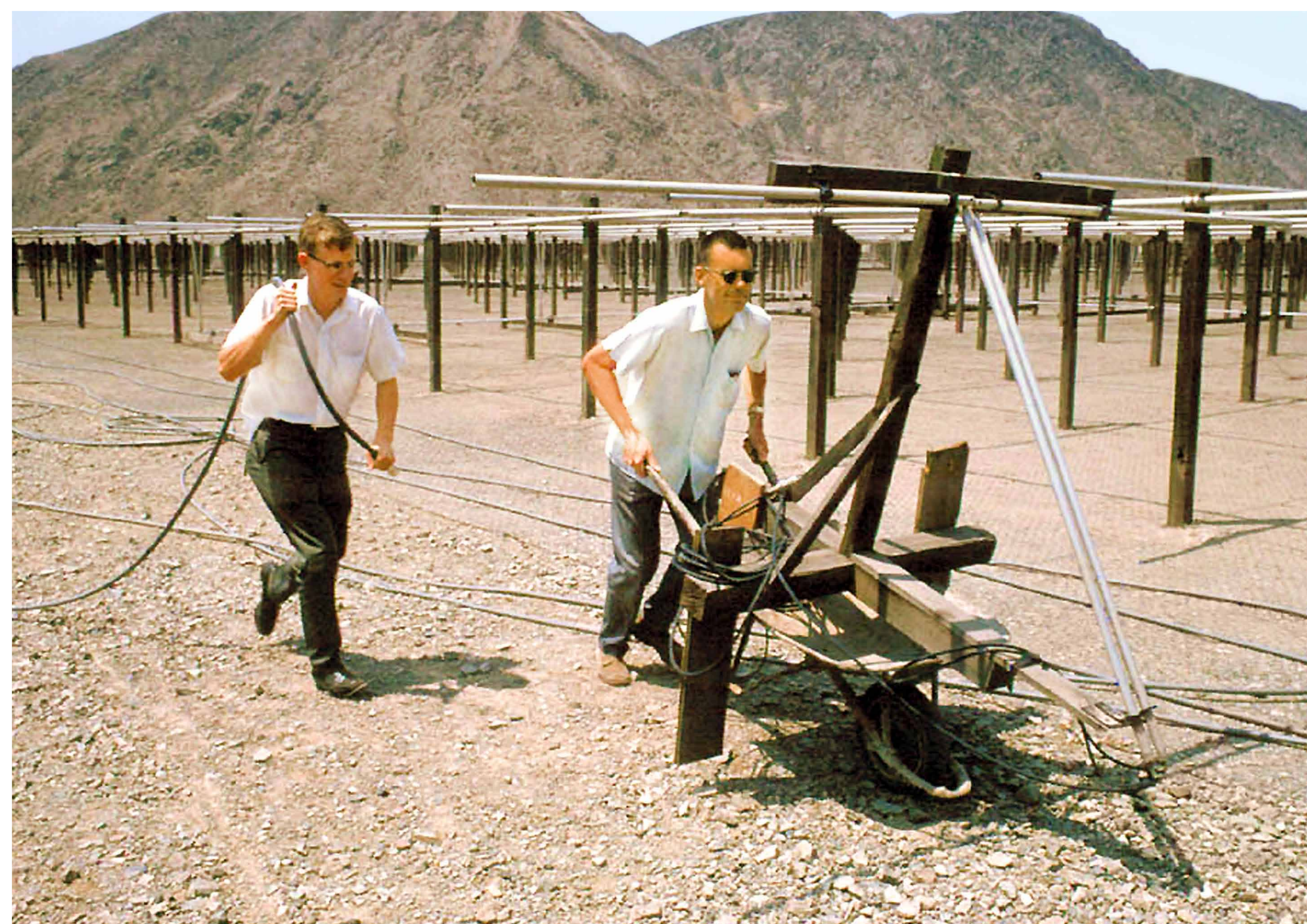
Staff in action: In 1966 at UCSD we were preparing to build three widely separated array antennas for use in measuring drift characteristics of the Solar Wind using signals from radio stars.
